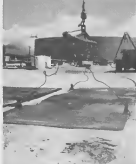
SHEETS ARRIVE for the replacement tank and are laid out so that they may be prepared and worked on before installation.
